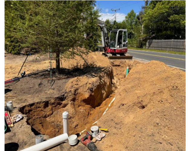
Preparing to backfill
