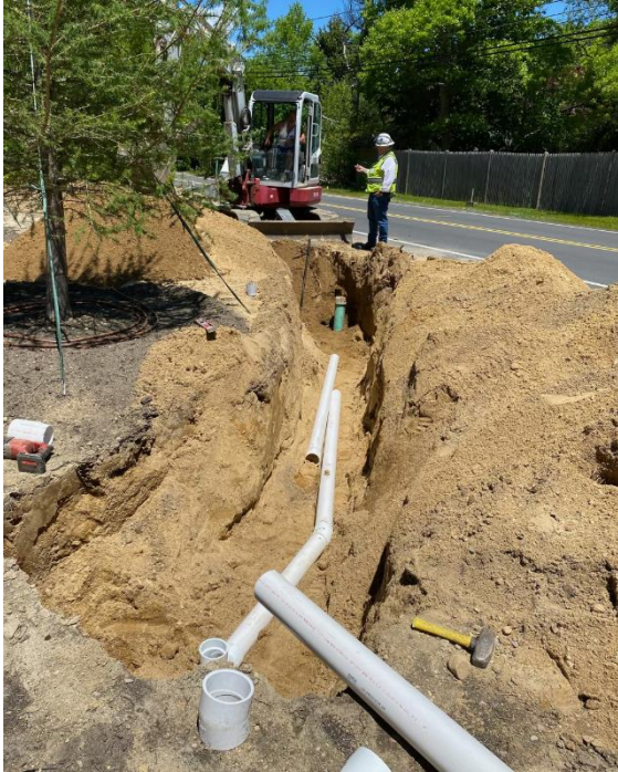
Excavation and connection layout, accompanied by DPW inspector
